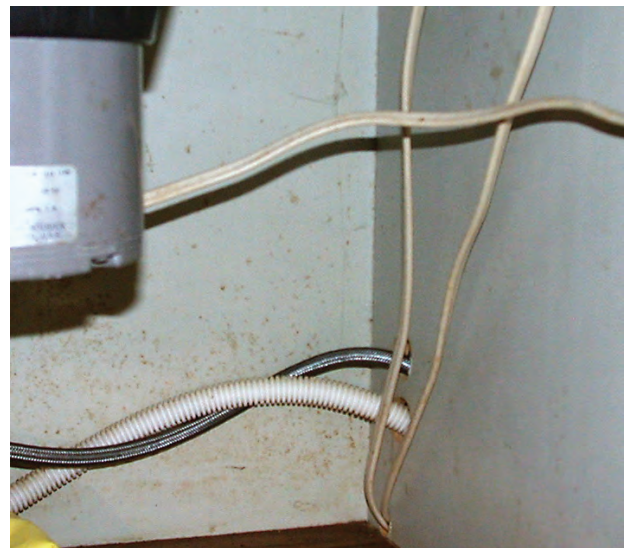
Visible Aspergillus mold growth in kitchen-sink cabinet May Indoor Air Investigations LLC
